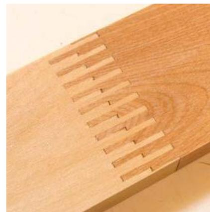
This joint can be modified to be different shapes for any aesthetic style.
