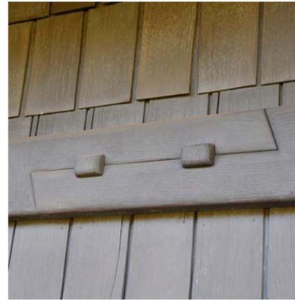
This joint has two cogs for extra support against tension.
