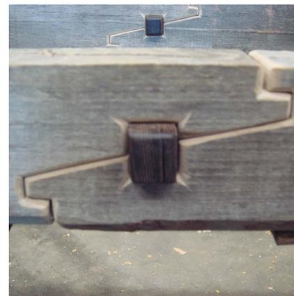
Scarf Joints can be made at an angle, or parallel to the edges of the piece.
