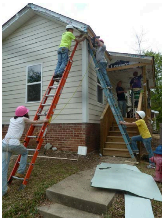
Figure 1: Our Collegiate Challenge group 2012 attaching siding to the house.
